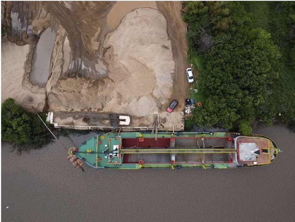
Figura 2.6.1-2: Draga SC Dredger.
